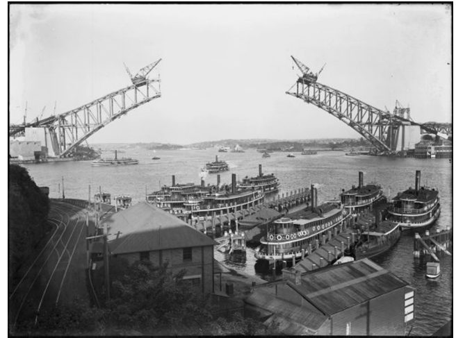
Fig. 4. The Sydney Harbour Bridge under construction from both ends (Photo credit: National Library of Australia, nal.pic-vn3071984-v).
